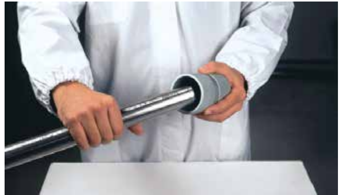
Figure 6 - Deburring the pipe
